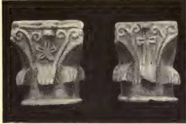
Fig. 190.—San Giorgio in Valpolicella. Church. Capitals of Ciborium (712-740).
